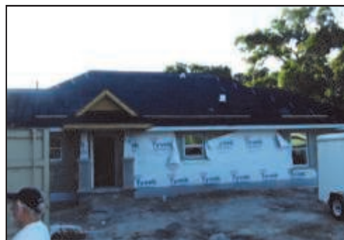
The Habitat House is well under way!
