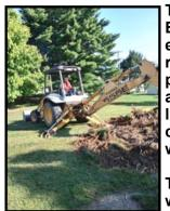
Thanks to Richard Blackstone and his equipment we were able to remove the stump at the parsonage that was causing a root problem in the sewer line and causing some concern with the basement wall.
